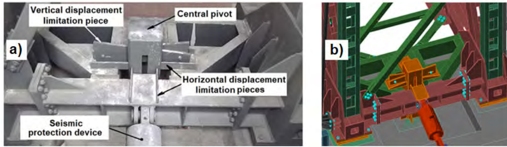
Figure 3. Metal block for displacements blocking (Tower T3): a) Photo image; b) Rendering
