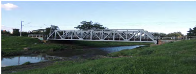
Figure 1: View of the bridge
