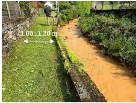
Figure 1: Existing street carriageway and valley (km 0+220 – km 0+270)
