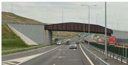
Figure 1: National road DN 1 over the A10 highway
