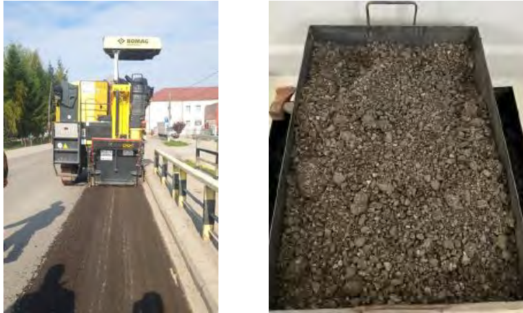
Figure 1: Reclaiming asphalt pavement and sample preparation
